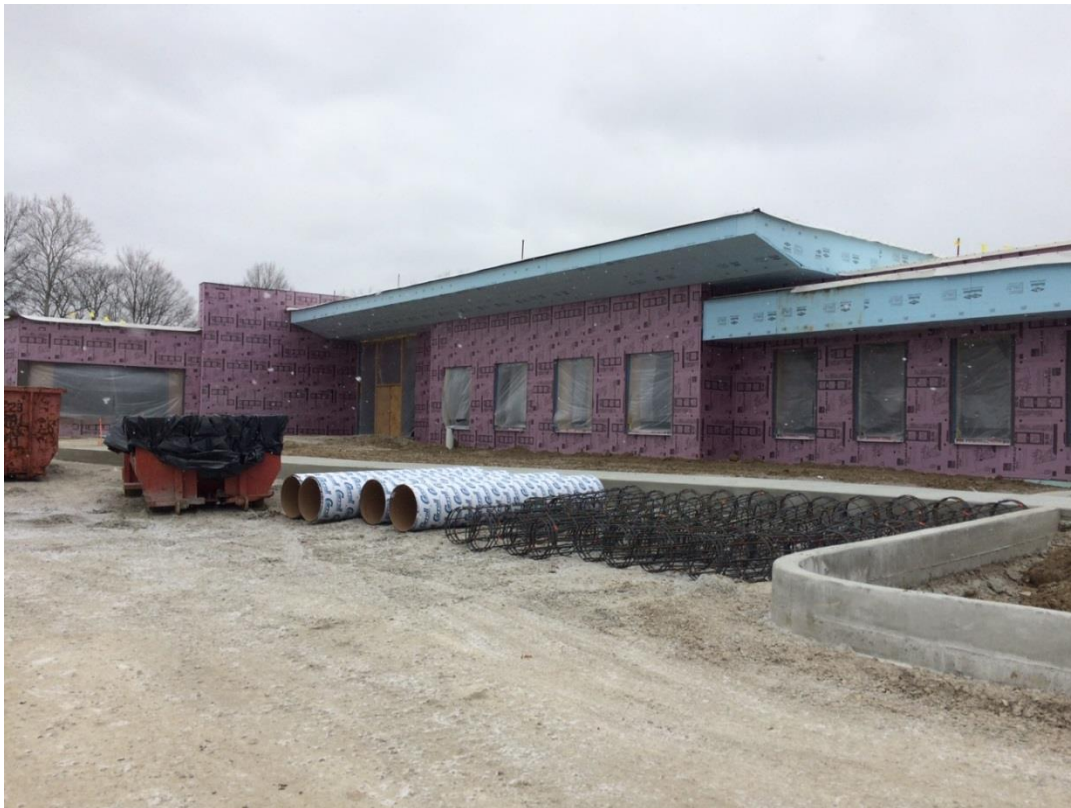
Project Site on January 9, 2019 View of the entrance with the parking lot light pole foundation cages.
