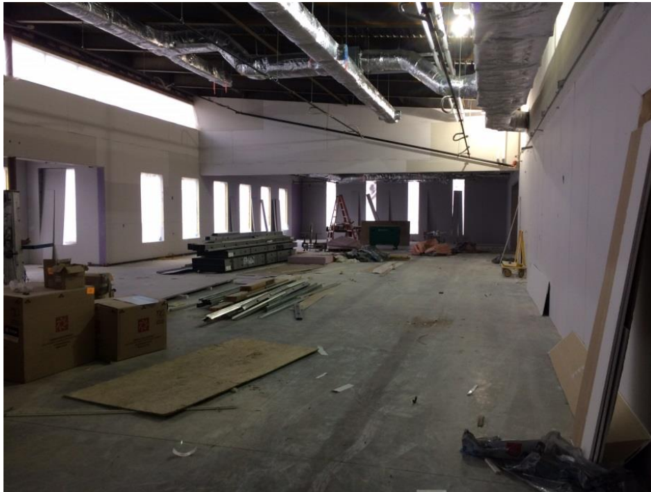
Project Site on January 9, 2019 View inside looking east showing the Children's area.
