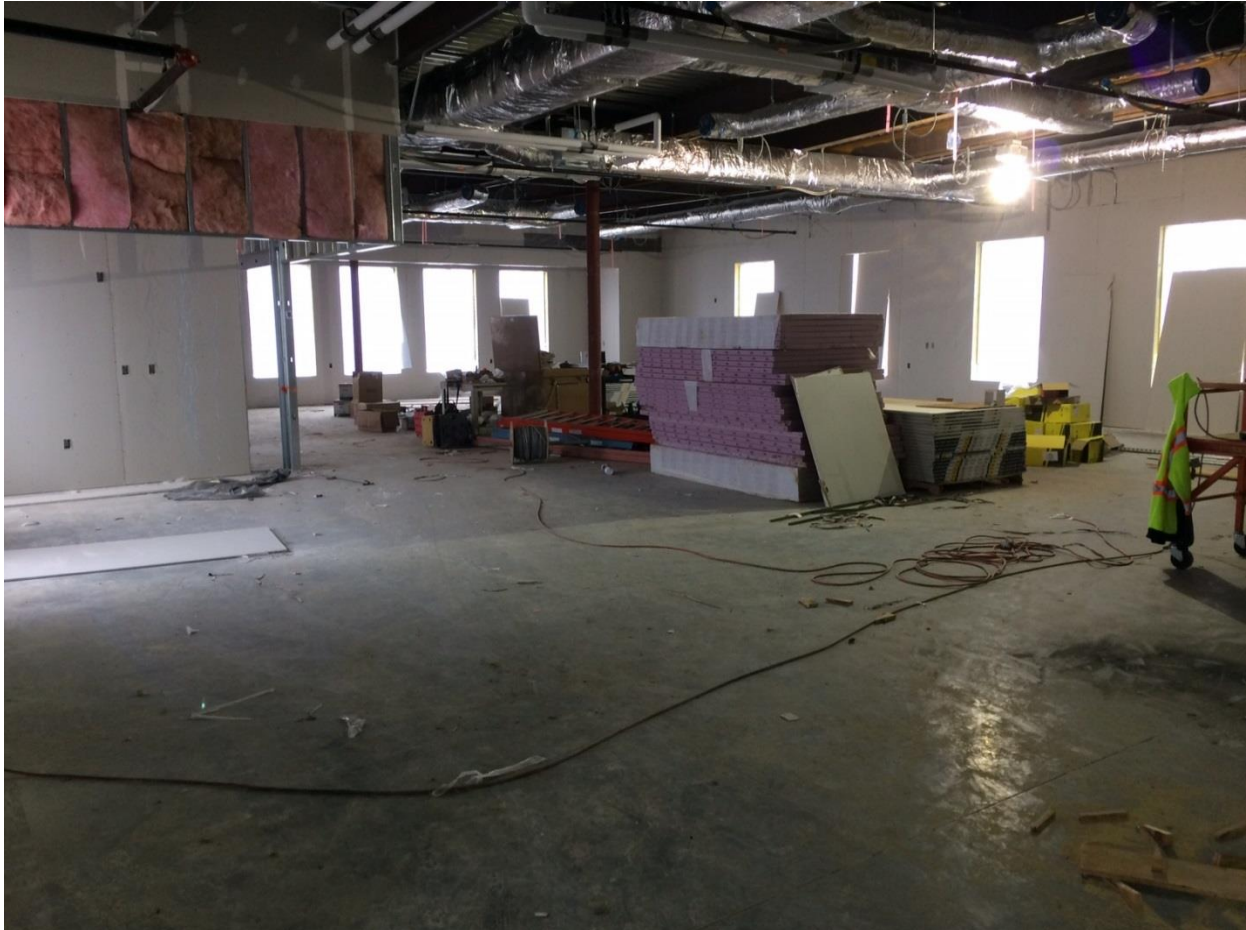
Project Site on January 9, 2019 View inside looking north showing the Adult's area.
